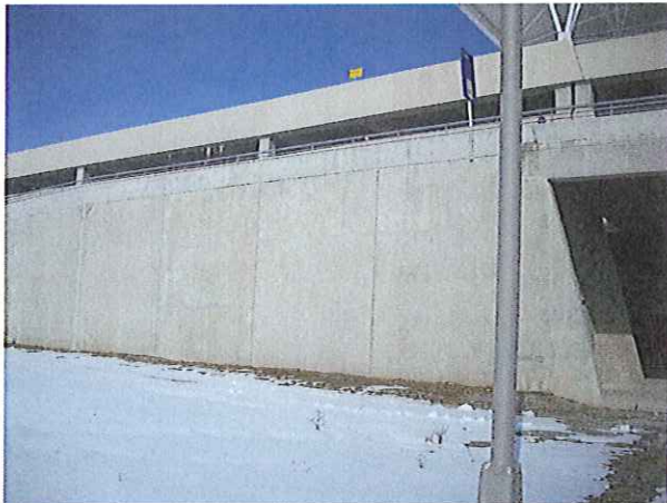
North Speed Ramp & North Storage Room
